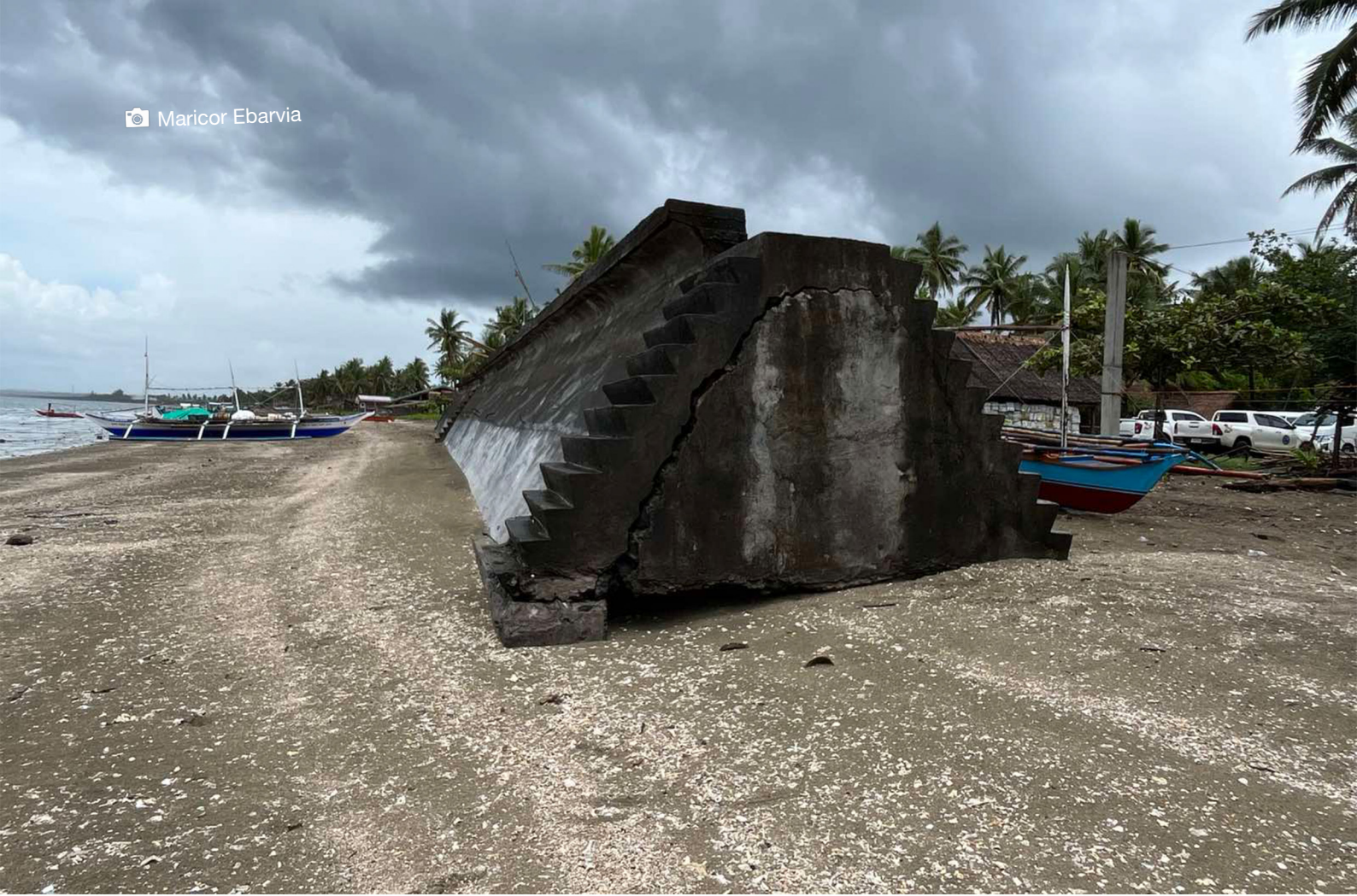
Partially built seawall in Pilar, Sorsogon
